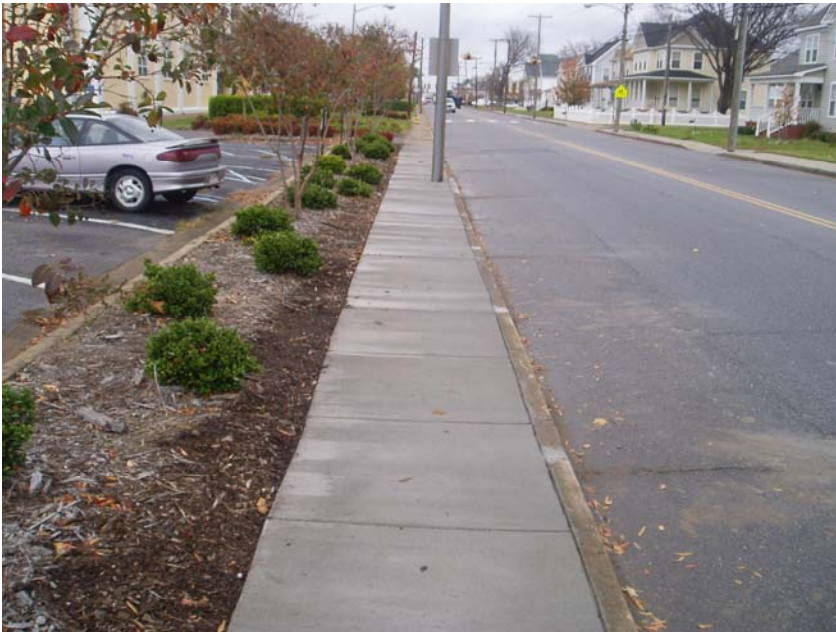
New Sidewalk on South Main St.
