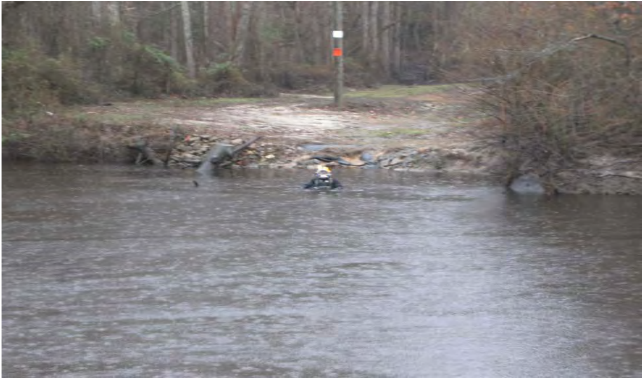
Diver standing on 30" pipeline at the west bank of the river.
