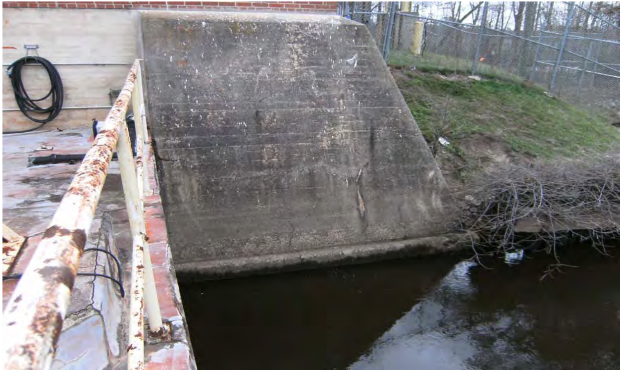
View of west face, south end above the scoured area.
