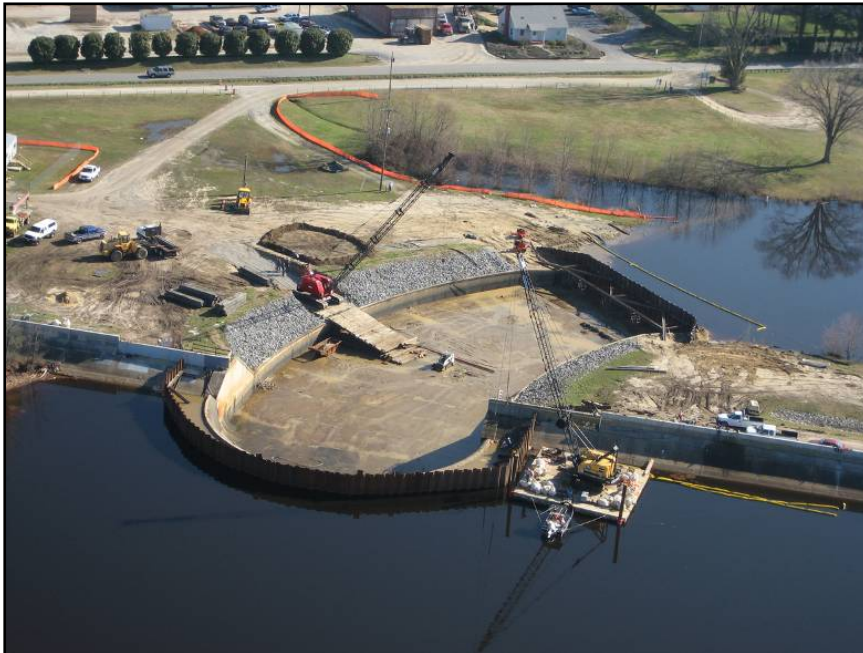
Lake Burnt Mills Dam during construction and rehabilitation.
