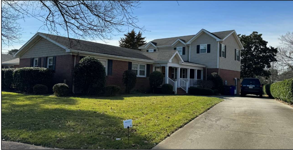
979 Anna Street, northeast oblique. This was one of the houses originally oriented with its side elevation facing the street. The two-story section is an addition that took the place of an attached garage and the original roof on the house was changed from a hipped roof to a gable. Photo by the author, February 2024.
