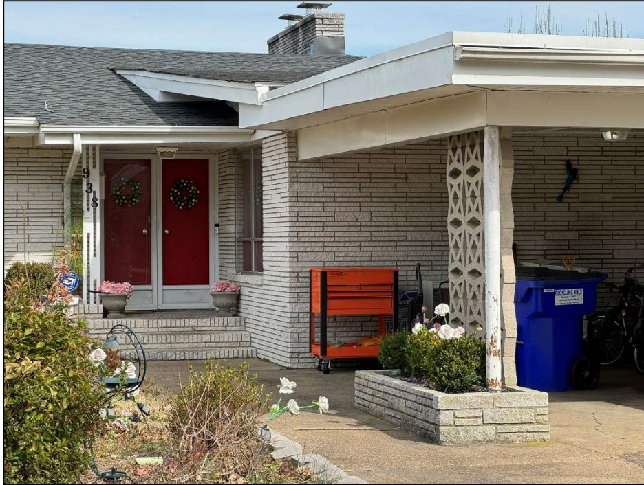
938 Anna Street, entrance detail, note breeze block screen supporting the original carport roof on the right and the midcentury modern-style post supporting the entry porch roof on the left.
