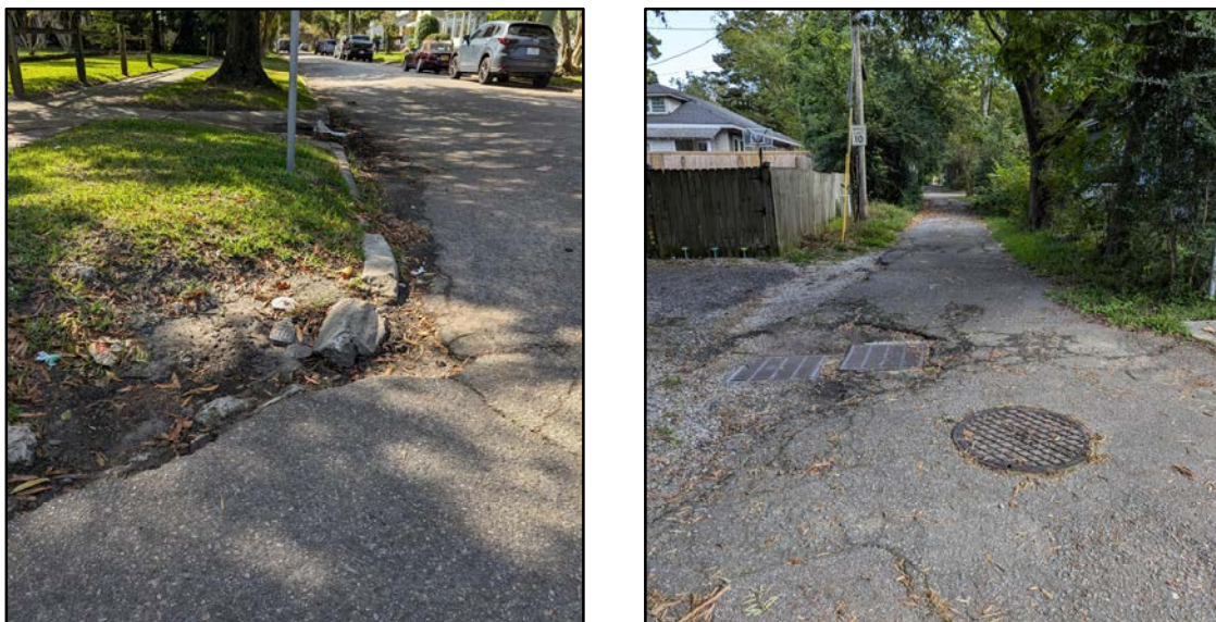
Figure 33: Erosion and Degradation of Curb (left) and Drainage Inlet (right)
