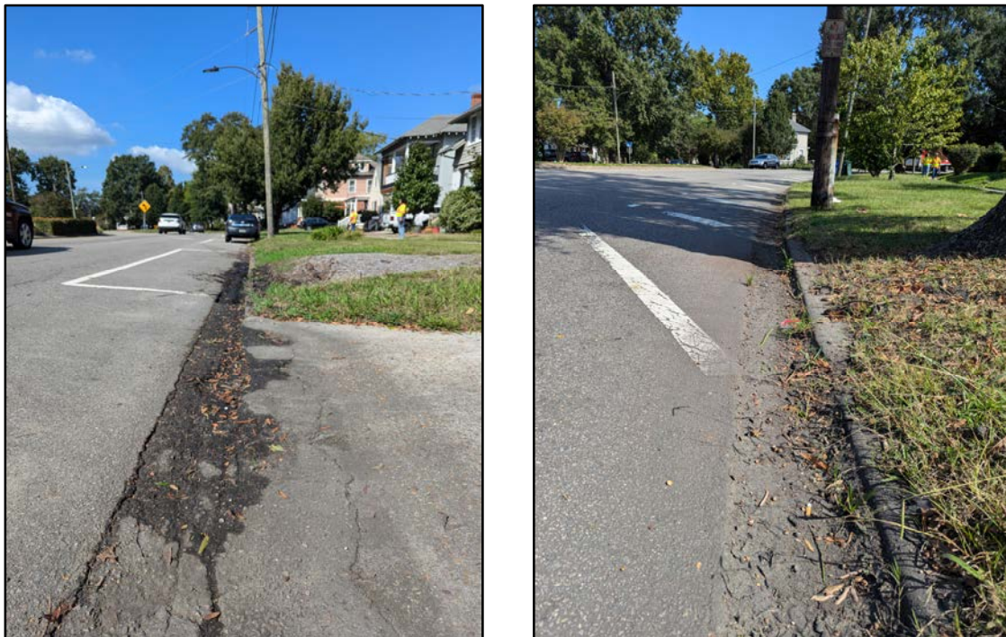
Figure 33: Erosion and Degradation of Curb (left) and Drainage Inlet (right)
