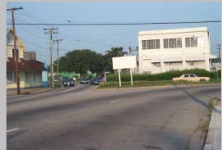
Electric Sub-station on Lafayette Boulevard
