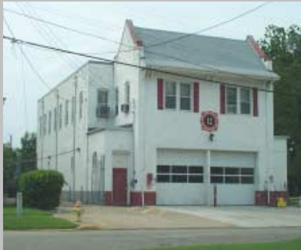
Fire Station #11 on Verdun Avenue
