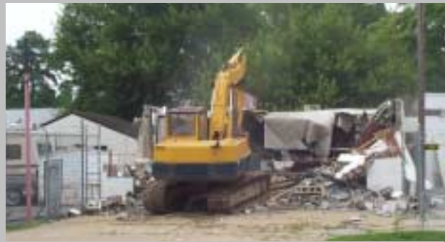
2605 Lafayette Boulevard Demolished on July 23, 2003
