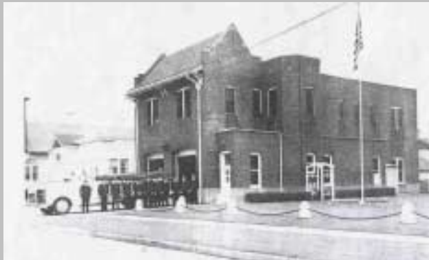
Fire Station #11 on Verdun Avenue
