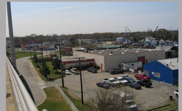
Existing conditions at the Campostella Bridge west site.
