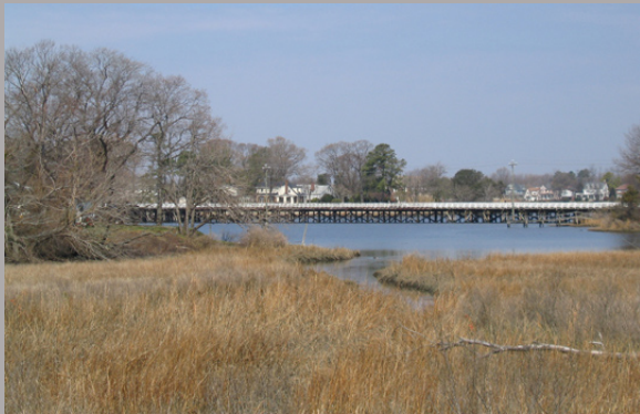
Steamboat Creek Bridge is currently closed to vehicular and pedestrian traffic.
