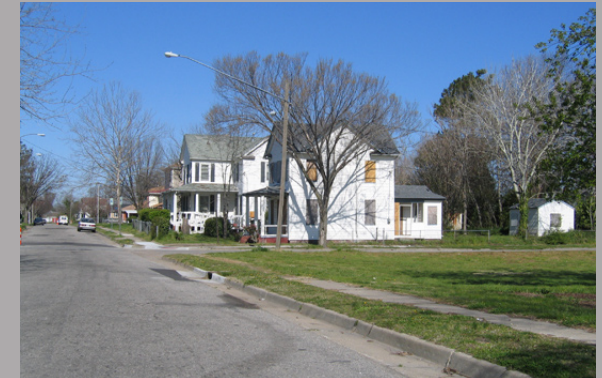
Vacant/open parcels offer opportunities for new construction in the Campostella neighborhood.
