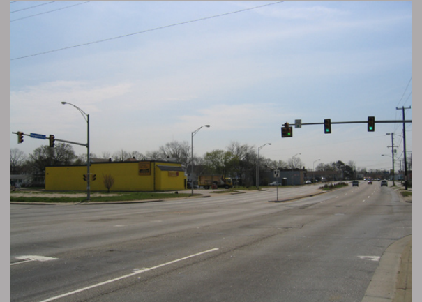
Stamped asphalt crosswalk at the intersection of Filmore Street and Campostella Road.
