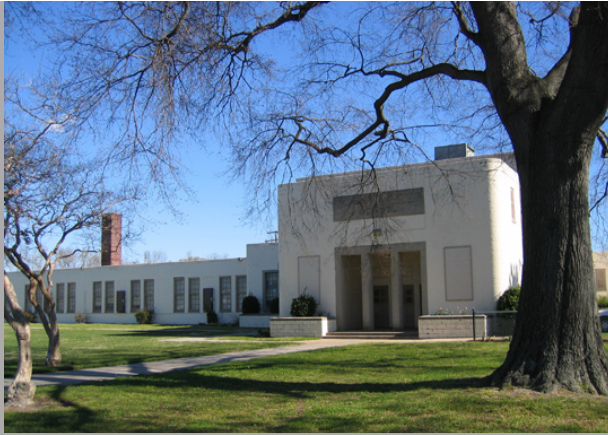
Opportunities exist to redevelop the former Tucker Elementary School site for recreation uses.
