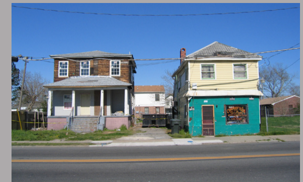
Blighted structures along Wilson Road.
