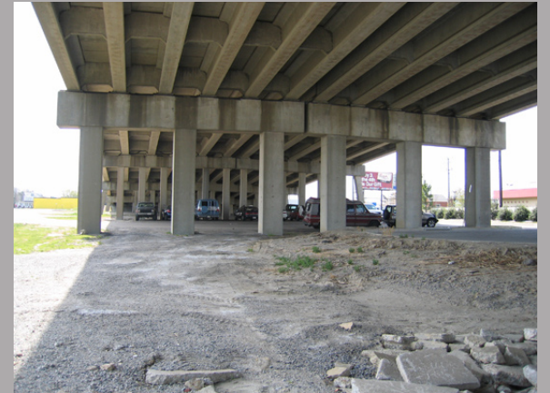
Existing pedestrian access under the Campostella Bridge.
