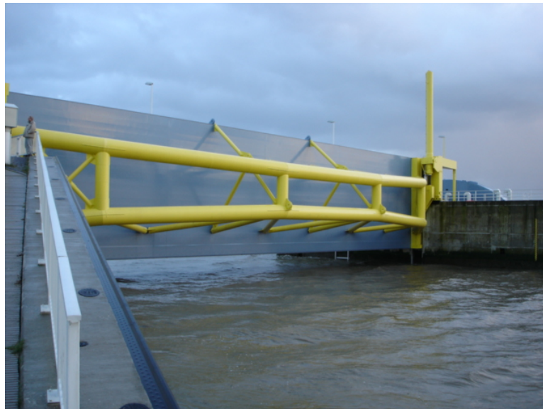
Ems Barrier lift gate (Source: Hein Mück, Wikimedia Commons)
