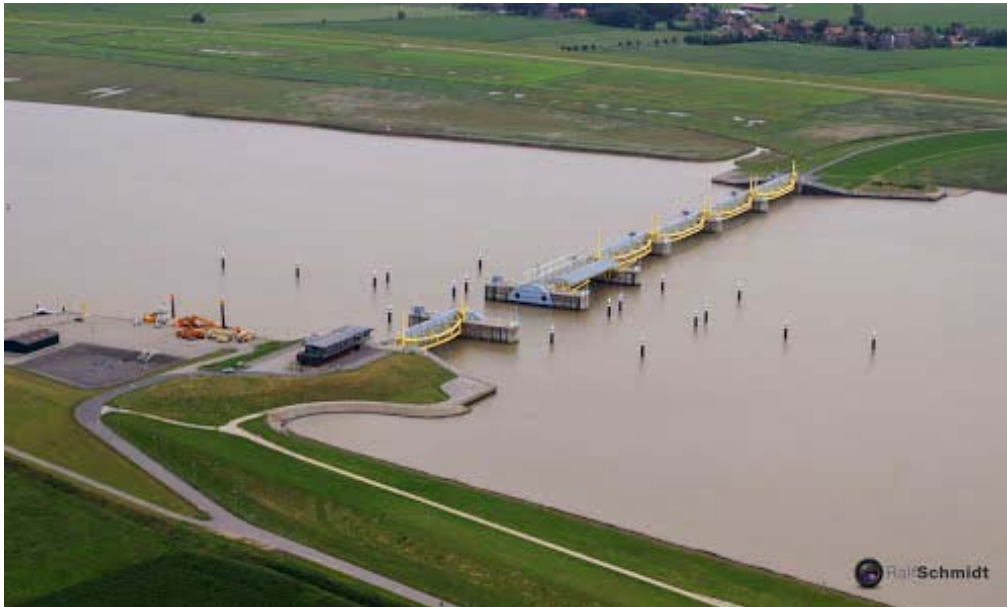
Ems Barrier, Germany northern aerial view. Constructed between 1998 and 2002, which includes three different gate types:
