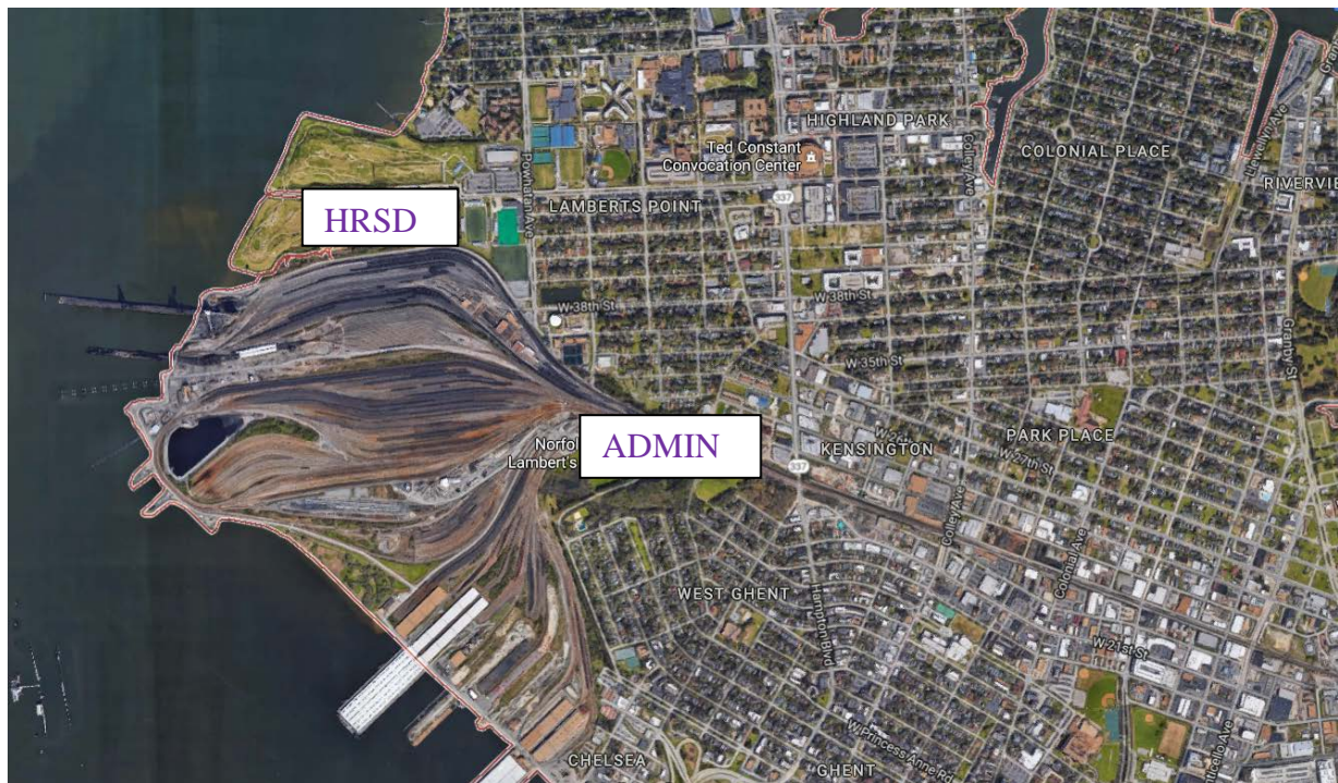
HRSD = HRSD monitoring station. ADMIN = ADMIN monitoring station
