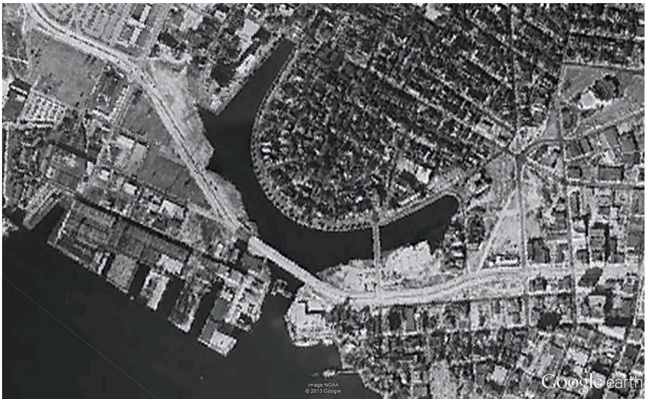
Photo 6: Circa 1964 Aerial showing probable wetland fringe along southwestern shoreline of the Hague (source: Google Earth Professional)
