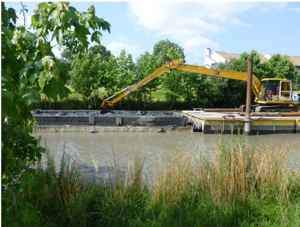
Photo 2: Small mechanical dredging operation.
