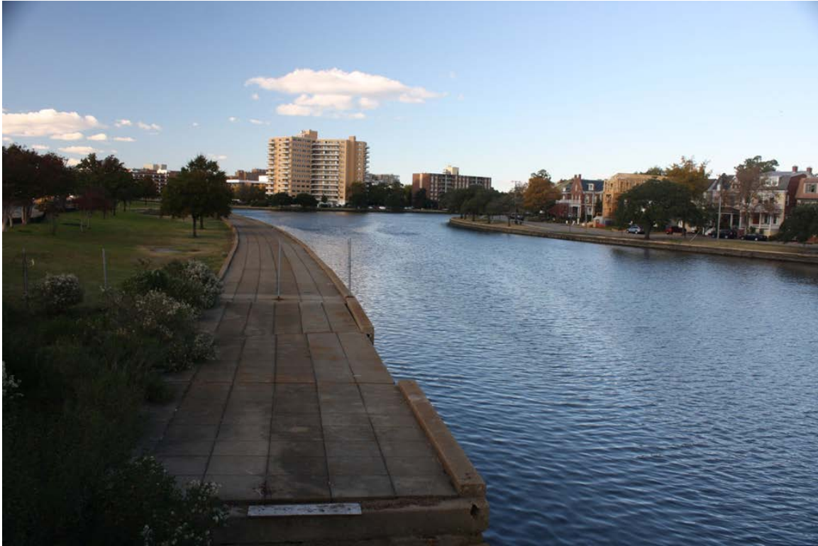
Photo 7: Potential site for living shoreline fronting promenade west of the Brambleton Ave bridge
