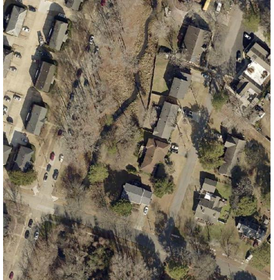
2018: After Construction - Single Restored Channel
