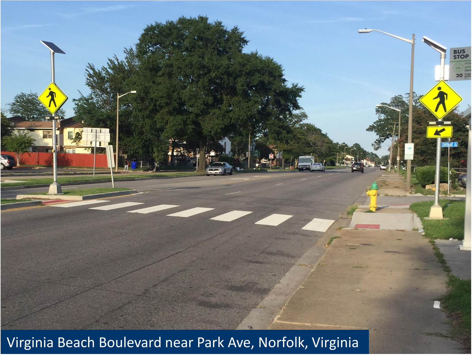
3. Rectangular Rapid Flashing Beacons
