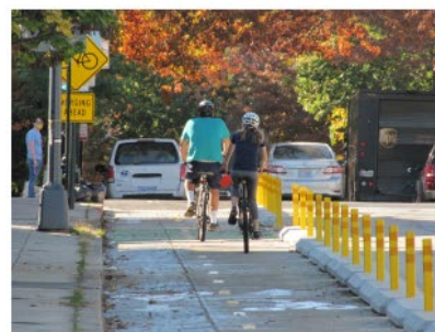
Flex posts with precast concrete curbs
