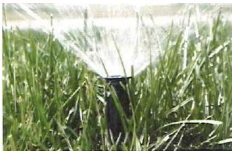
Due to the environmental hazards found on lawns, irrigation systems are considered high hazards with potential to backflow into the public water distribution system. For this reason, these systems must have an approved backflow prevention assembly installed and tested annually. It is the owner's responsibility to ensure that cross connections do not exist, and that the backflow prevention device is installed and maintained.
