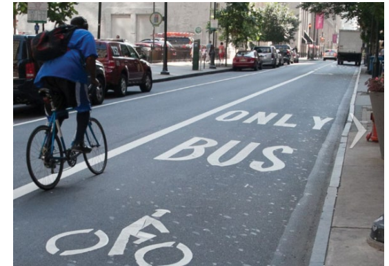
A combined lane for buses and bicyclists, such as this one in Philadelphia, PA, is one possible design approach. Image Source: NACTO
