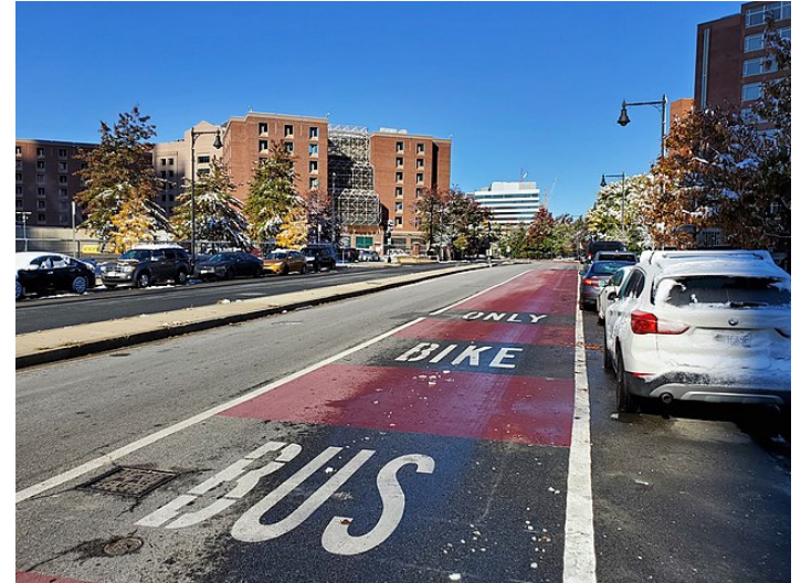
Roadway striping for a combined bus and bike lane. Image source: Wikimedia Commons
