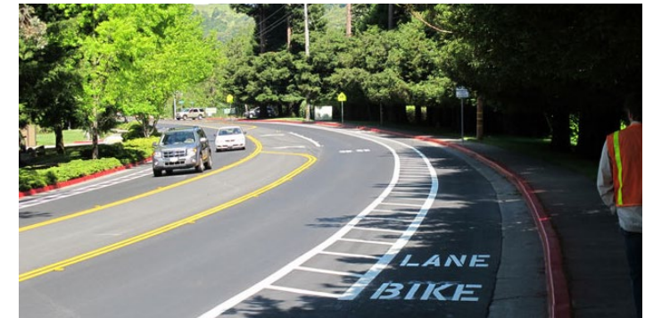
A conventional bicycle lane is a bicycle lane that is not vertically separated from vehicle travel lanes. Conventional bicycle lanes may be directly adjacent to the vehicle travel lane or may have a painted buffer. Fairfax, CA. Image Source: NACTO
