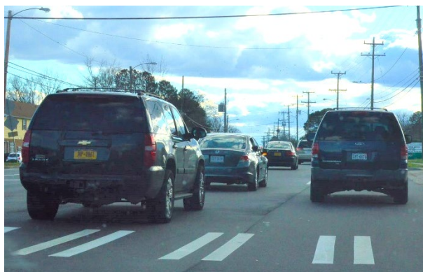
Bar Pairs are a common crosswalk marking type in Norfolk.
