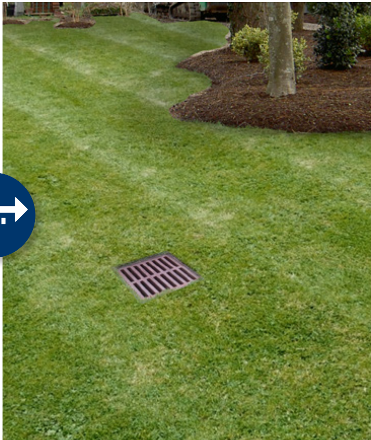
DRAIN CONNECTED TO UNDERGROUND PIPE
