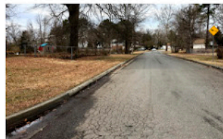
Very few storm drains—primarily reliant on above ground flow and infiltration into private yards.
