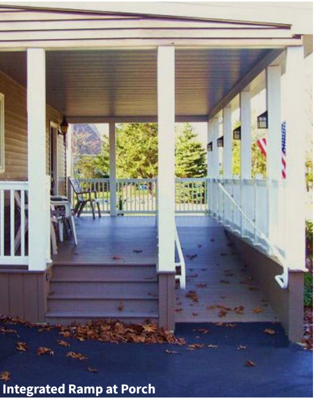
Integrated Ramp at Porch
