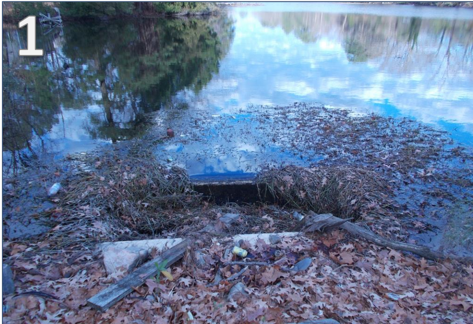
Existing debris filled outlet structure at Meadow Lake
