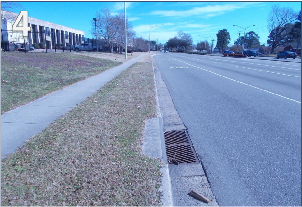
Existing catch basin on north side of VB Blvd.
