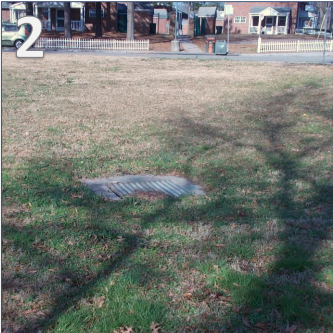
Drop inlet at northeast corner
