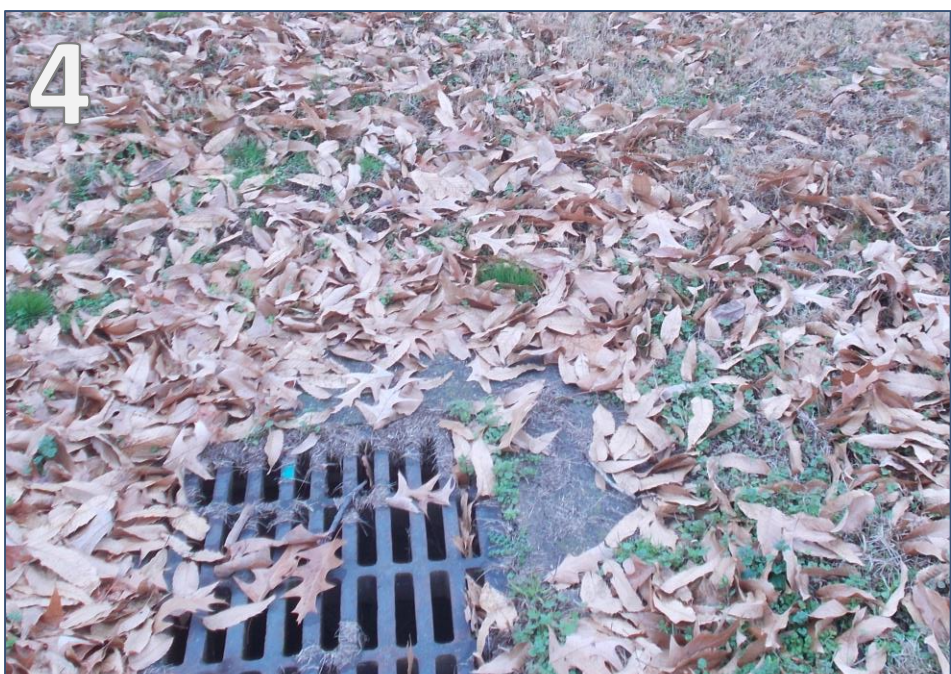
Drop inlet structure in right-of-way
