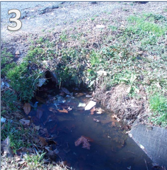
Ditch culvert connection
