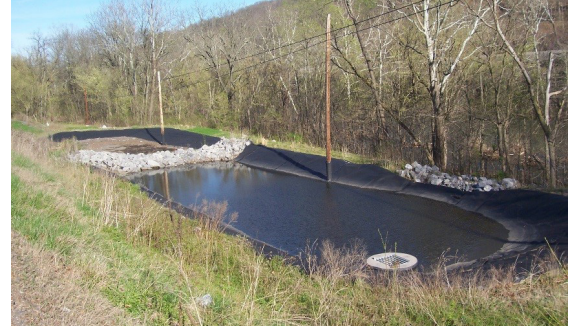
Temporary Stormwater Sediment Basin
