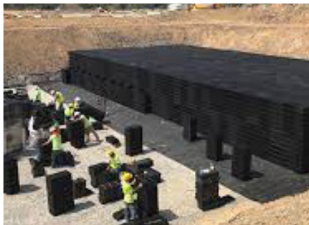
Modular Subsurface Detention R-Tank, ACF Environmental
