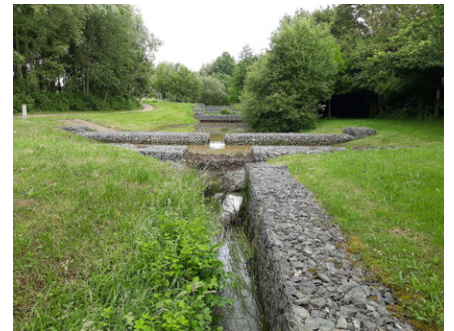
Gabions Reinforce Edge Of Waterway credit
