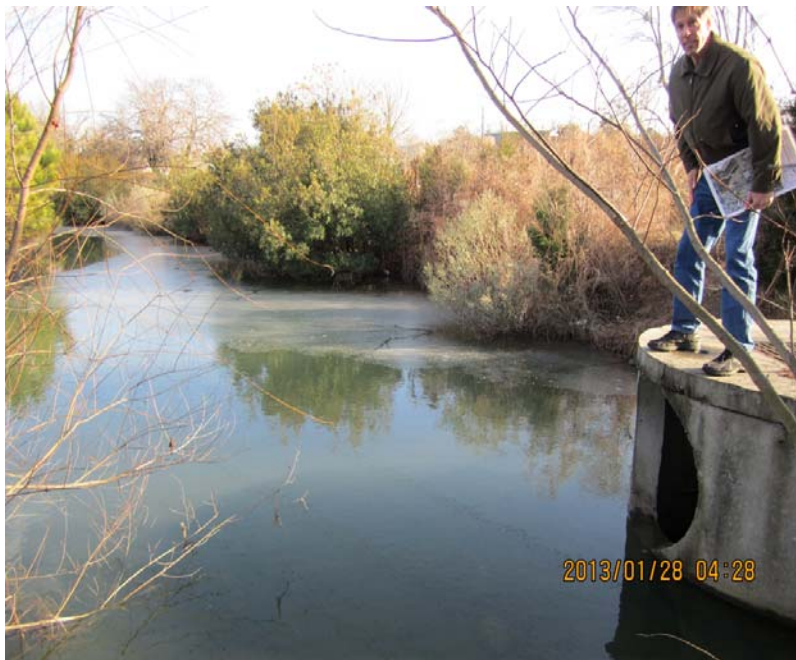
Figure 2-7 Central Business Park (Site ID 99-3931) – View of wet pond and principal spillway riser, looking east.
