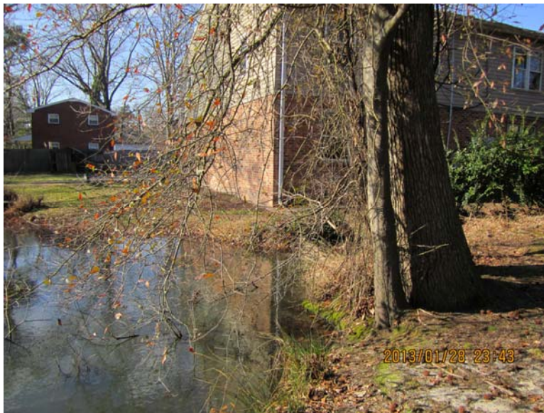
Lake Modoc (Site ID S6) – View of adjacent apartment building with a finished floor elevation approximately 12-inches above the normal pool.
