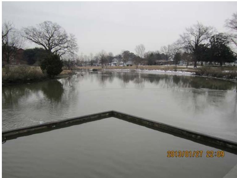
Ballentine Elementary School Lake (Site ID S2) – View of wet pond with concrete weir and orifices around principal spillway.
