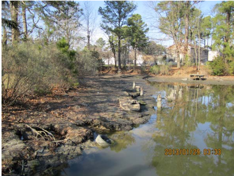
Meadow Lake (Site ID S15) – View of southwest portion of the upstream dam slope, which shows the reduction in normal pool level & sediment accumulation.
