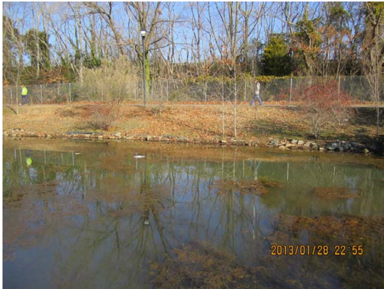
Norview High School (Site ID 02-0010) – View of wet pond with heavy algae growth, looking north.
