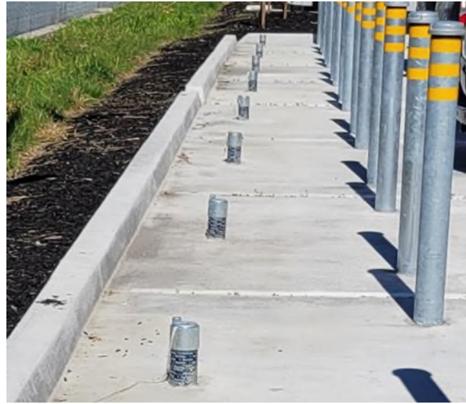
Figure 37. Example of stub-outs installed to add EV chargers in the future
