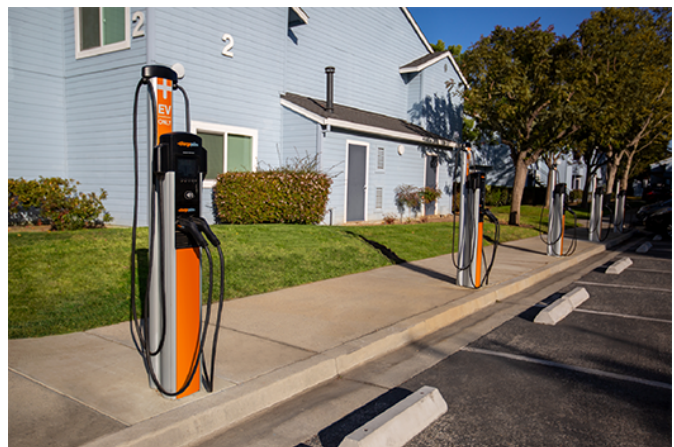
Figure 26. Example of MUD EV charging
