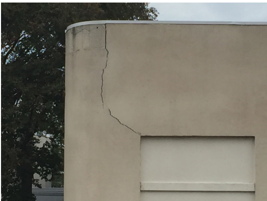
Typical stucco failure
